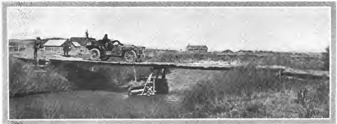
Typical Western Country Met with in Wyoming, Where Bridges Are to Be Crossed with Much Caution.
